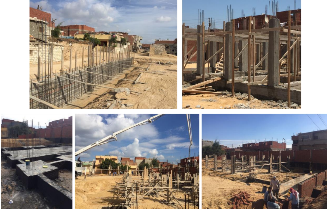
*Construction of the Youth Center in Alexandria
